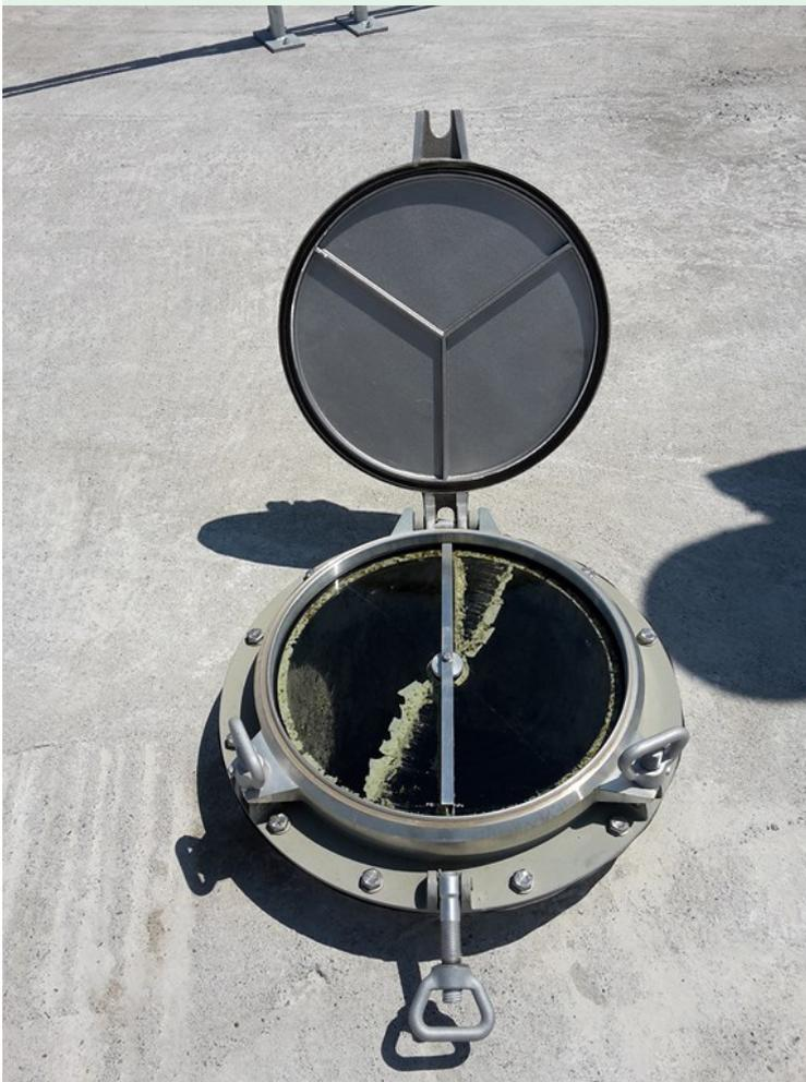
The AAT View ports are used to look inside various containers, tanks and shafts in biogas plants.
