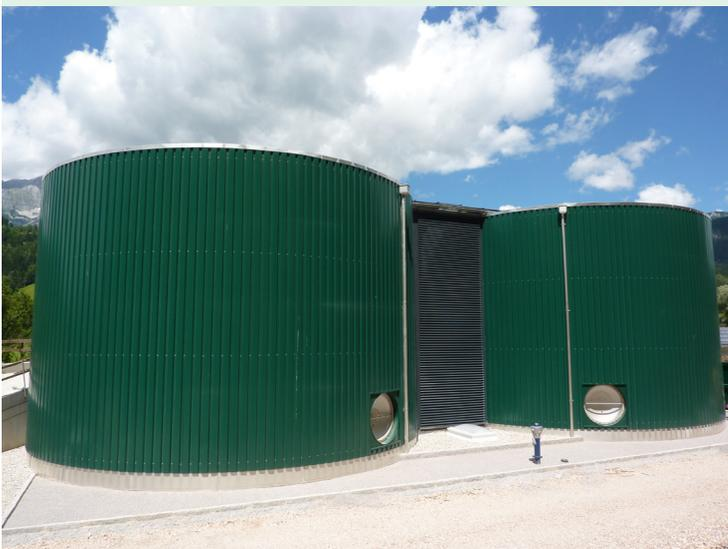
The AAT package plant digestion combines the sludge digestion and the gas storage in a simple and maintenance-free system.
